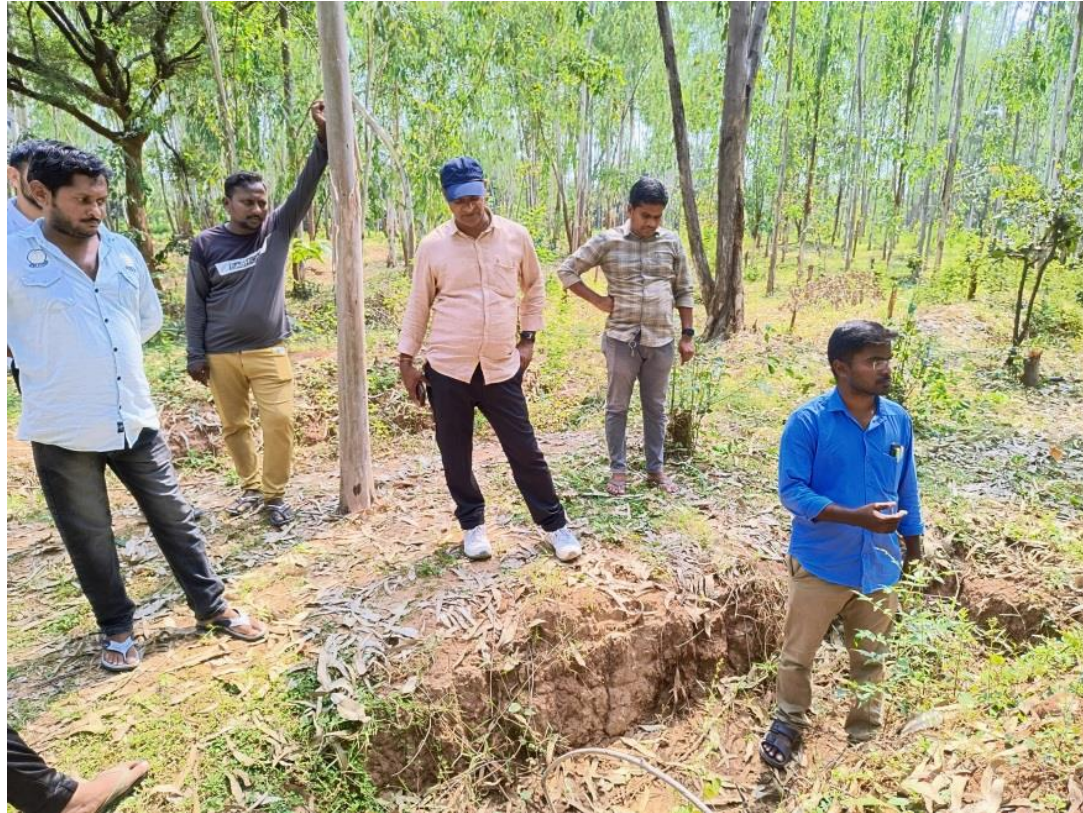
Digging of trenches for groundwater rejuvenation.
