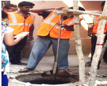
Step 2: Removal of Silt (manual)
