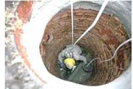
Step 3: Entering manhole in presence of field officer under inevitable situations.
