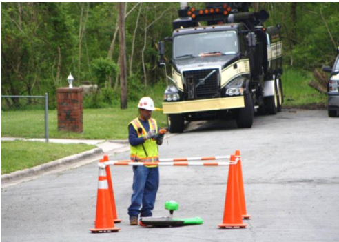
Step 1: Identify manhole to be cleaned
