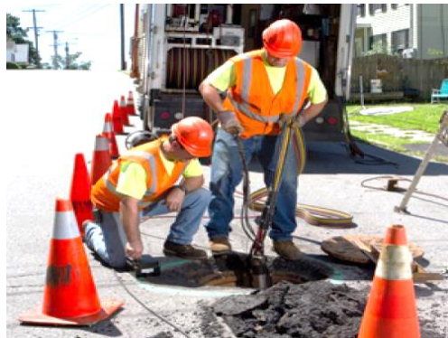
Step 4: Usage of sucking & jetting vehicle (Mechanical).
