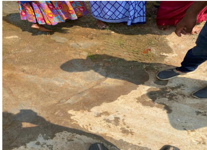
Mission Bhagiratha Leakage identification & Repair
